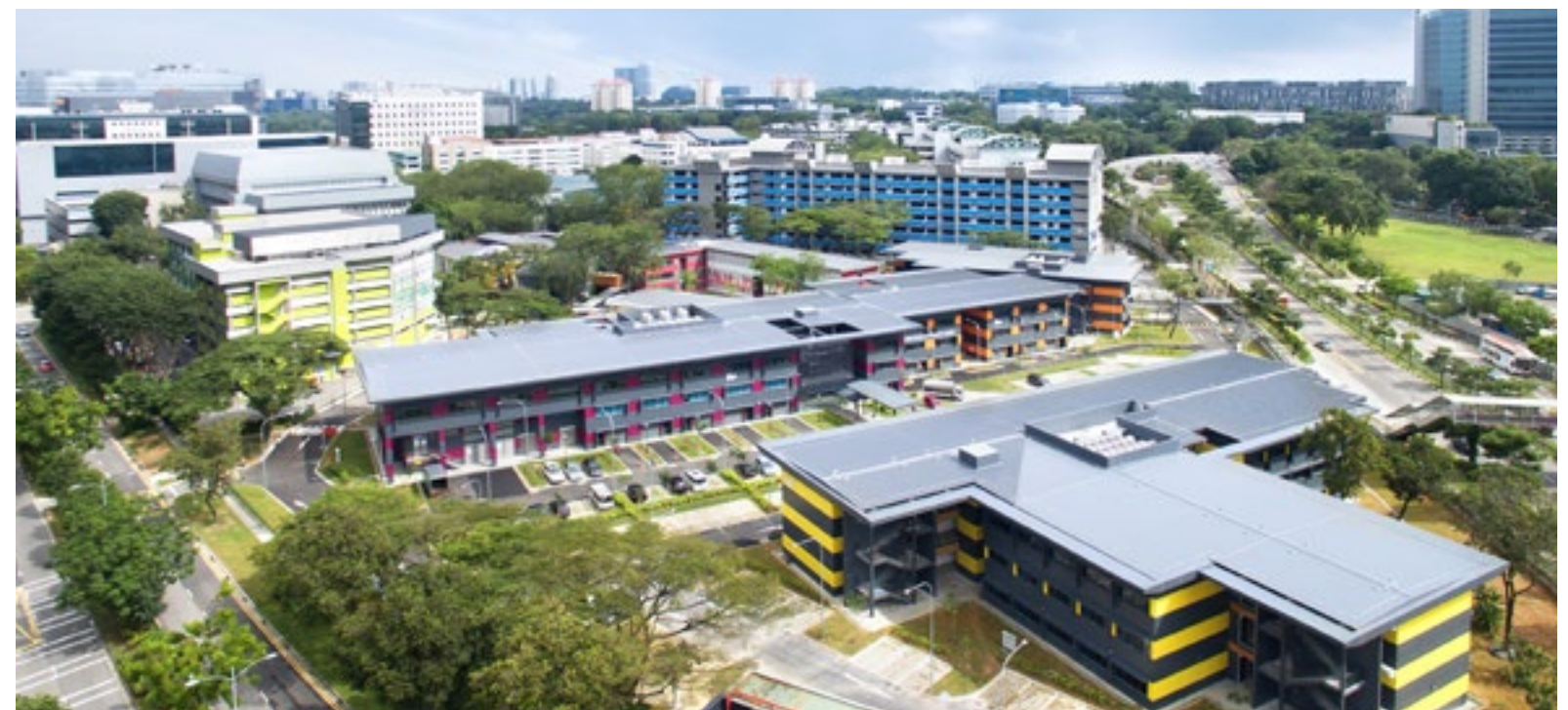
Top: In June 2022, Bombardier officially opened its newly expanded Singapore Service Centre in SAP, quadrupling its footprint from 100,000 sqft to approximately 430,000 sqft. This will allow it to support more than 2,000 business jet visits annually. Bottom: Over 700 start-ups can be found at JTC’s two LaunchPads.
