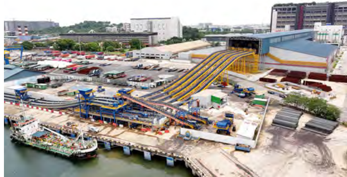
Above: Aerial view of the Ready-Mixed Concrete Ecosystem
