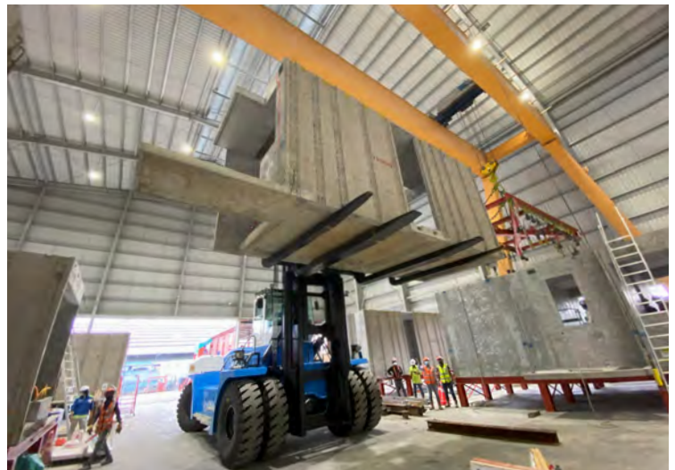
Below: Customised multi-functional 50 tonne forklifts for the lifting of PPVC.
