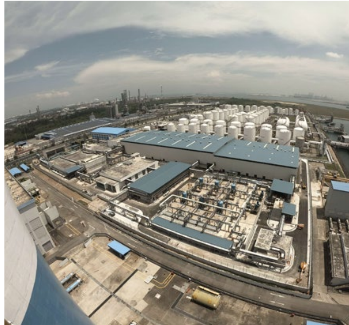
Equipped with the latest proven water technologies, the Jurong Island Desalination Plant is highly automated and requires at most three personnel to man. Photo courtesy of Tuas Power.
